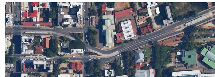
Figure 3.27 - One way BRT in Johannesburg, South Africa
