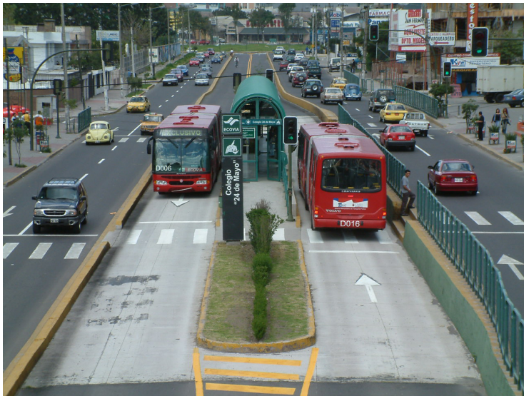
Figure 3.1 -Locating dedicated BRT lanes in the median ensures that they remain free of obstructions.
