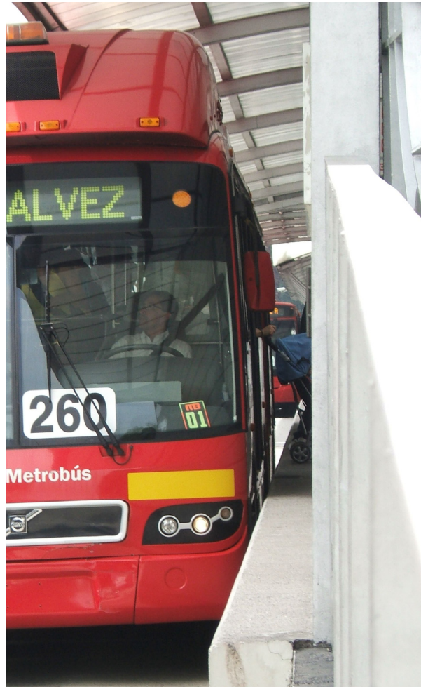
Figure 3.32 -Ledge extension at Metrobus BRT station in Mexico City to facilitate seamless boarding
