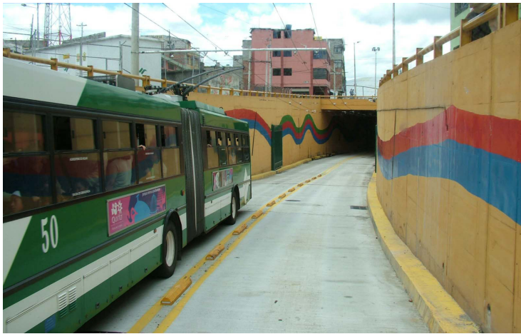
Figure 3.4 -A BRT underpass in Quito.
