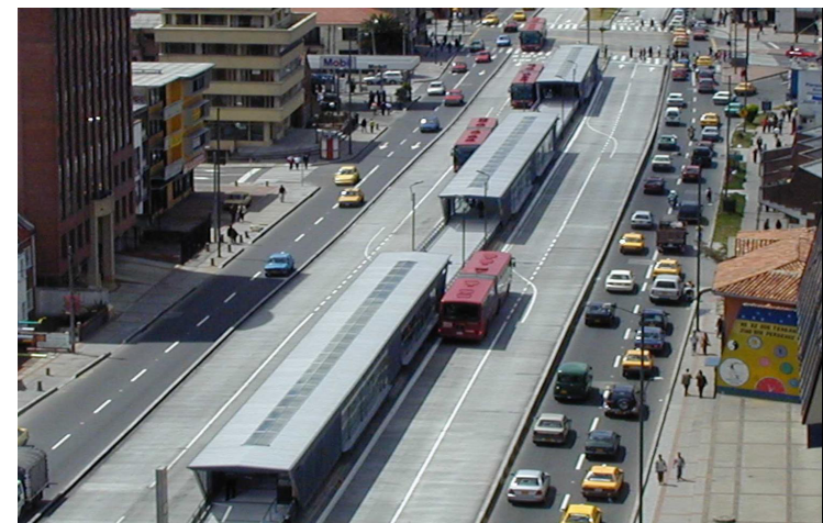
Figure 3.14 - Overtaking lanes and multiple stopping lanes increase capacity manifold
