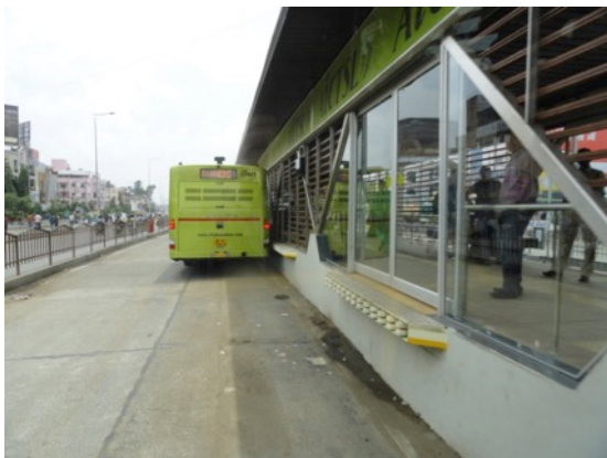
Figure 55: Cement concrete surface for BRT lanes and stations.
