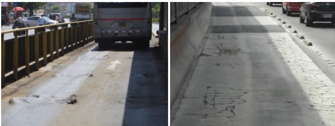
Figure 85: Effect of repetitive bus movements at BRT stations in Ahmedabad (left) and Mexico City (right).
