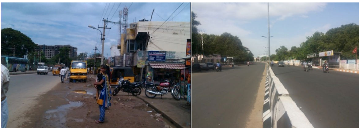
Figure 83: Existing pavement condition in Mettupalayam Road (left) and Avinashi Road (right).
