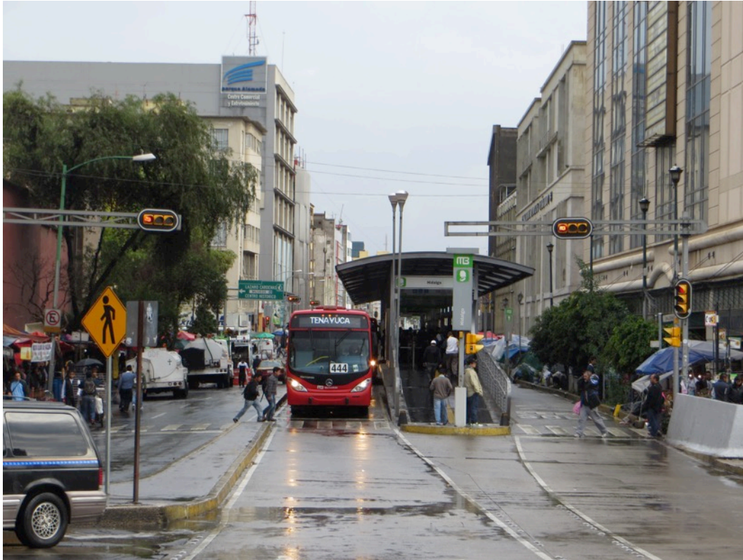
Figure 48: Physical planning includes the careful integration of buses, stations, street elements, and intersections designs.
