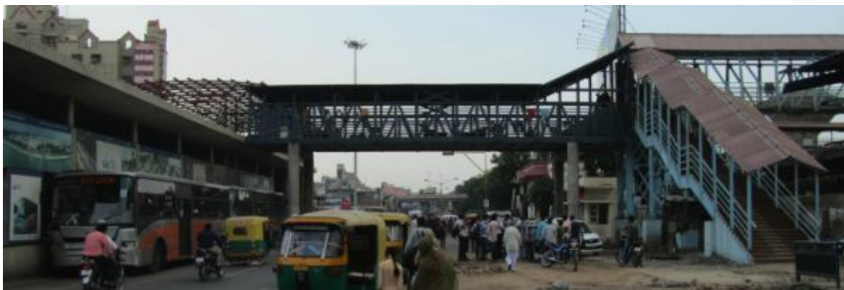
Figure 63: Connection between Janmarg BRT terminal (left) and Maninagar railway station (right), Ahmedabad.
