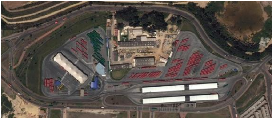
Figure 90: Co-located Bus depot and terminal of the Transmilenio BRT system, Bogotá (Google maps)
