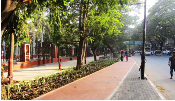
Cycle tracks should have asphalt/concrete surface finish. For even finish, paver blocks must be avoided on cycle tracks.
