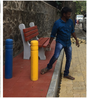
Tiles on pilot stretch
