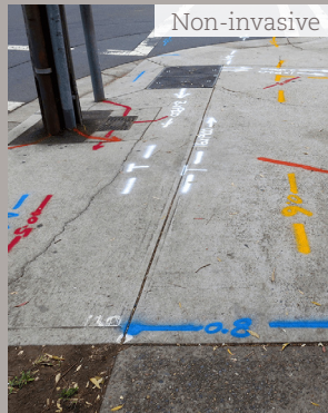
Marking utility positions on the road after GPR survey
