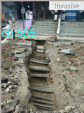
Trial pit for each chainage
