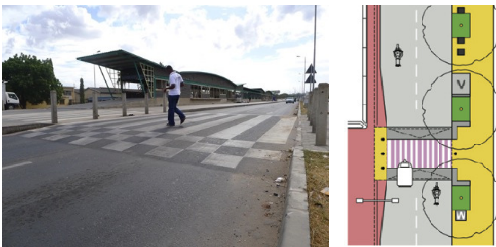
Figure 86: Access to midblock BRT stations should be provided through tabletop crossings at the same level as the adjacent footpath to improve accessibility.
