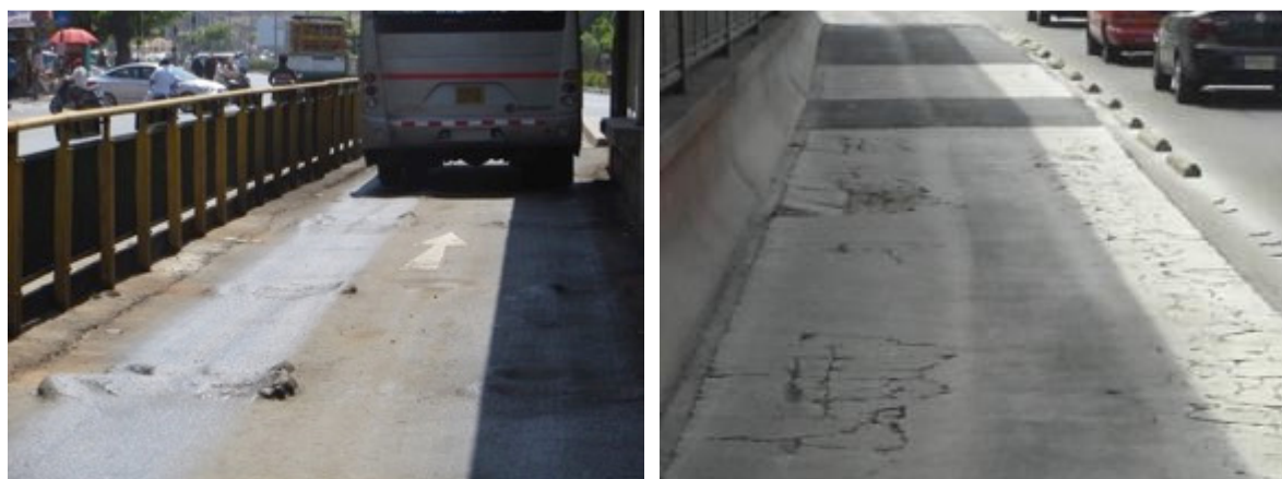
Figure 99: Effect of repetitive bus movements at BRT stations in Ahmedabad (left) and Mexico City (right).
