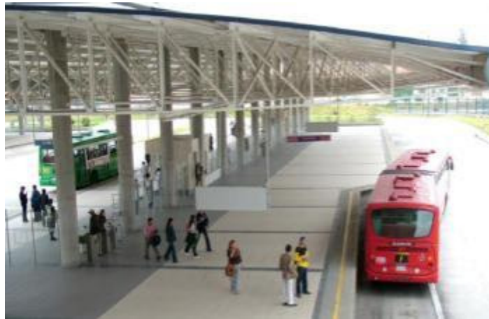
Figure 83: Transfer station between feeder and trunk BRT in Bogota, Columbia.
