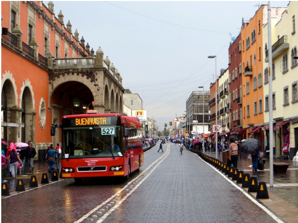
Figure 43: BRT can be implemented even on narrow streets, as demonstrated in these cross sections from Medellin (top) and Mexico City (bottom).
