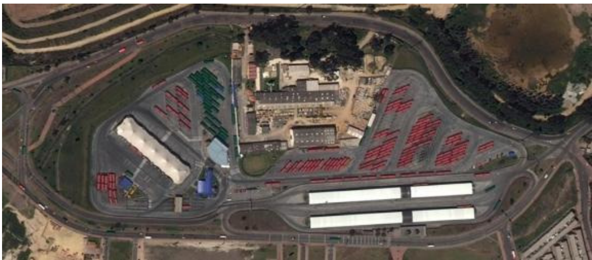
Figure 102: Co-located Bus depot and terminal of the Transmilenio BRT system, Bogotá (Google maps)
